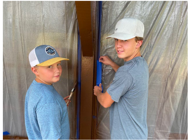
Jase & Tad Kinnunen Taping the Screens on one of the shelters.
